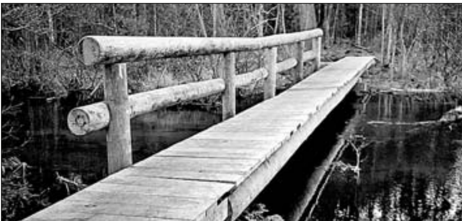
The bridge over Bigelow Creek built last year. PHOTO BY AARON PHIPPS
