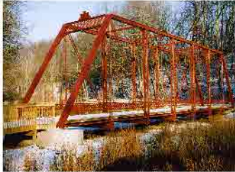
Restored Gale Road Bridge
